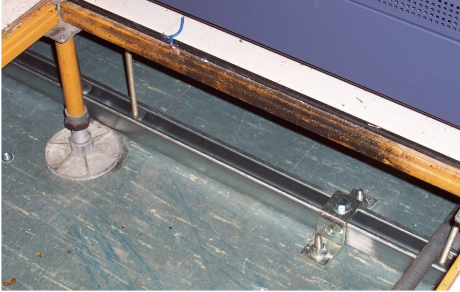
Figure 14-21 Illustration of Securing Cabinets and Racks on an Access Floor to a Concrete Slab Using Threaded Rod and Steel Channel
